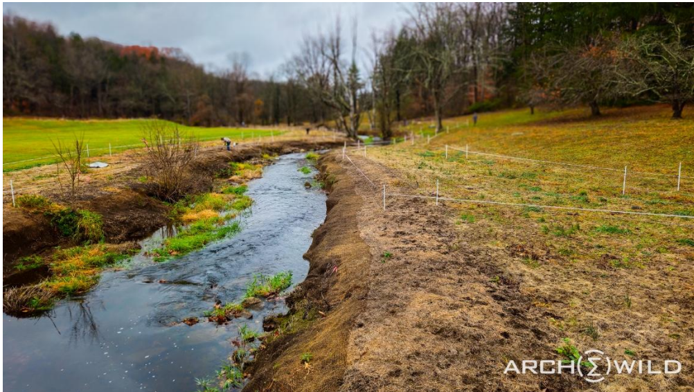
Figure 34 - Streamside meadow installations often require using techniques to hold seed in place during flooding events, such as coir matting along streambanks
