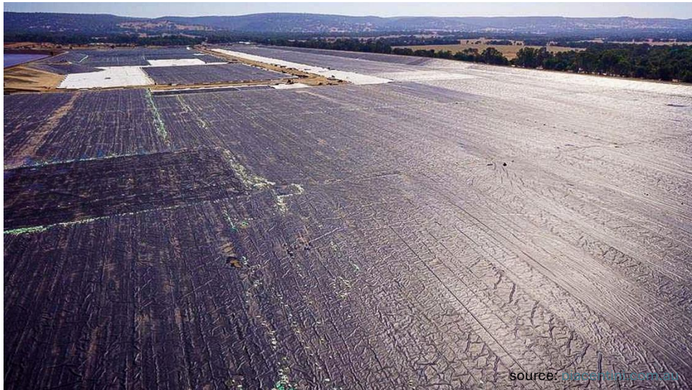
Figure 23 - Solarization of a meadow site can be performed and is occasionally successful, but takes a long time and can become quite expensive for large sites
