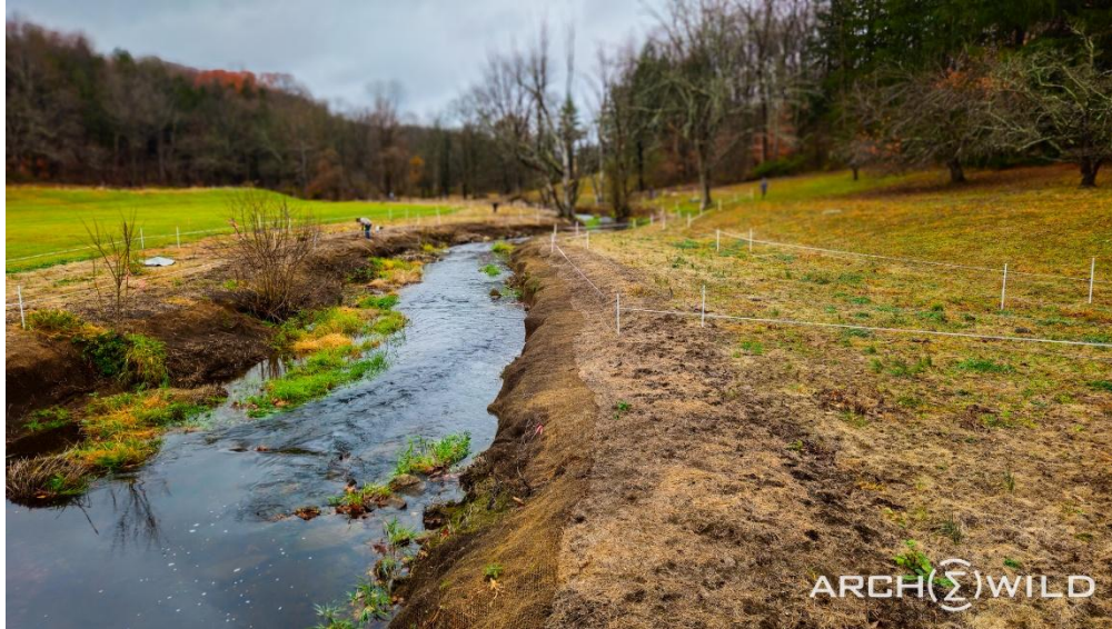
Figure 41 - Streamside meadow installations often require using techniques to hold seed in place during flooding events, such as coir matting along streambanks
